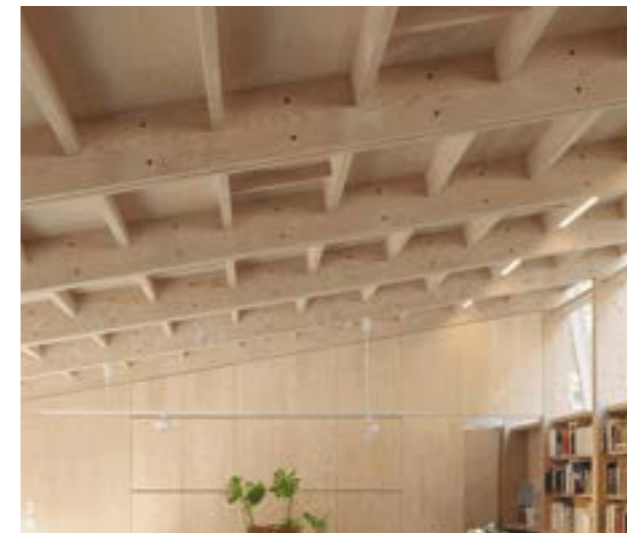
Interior - Simple plywood finishes with exposed beams and simple joinery
