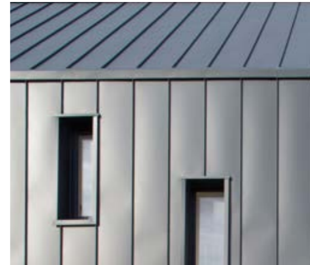
Roof & Canopy - preformed standing seam steel
