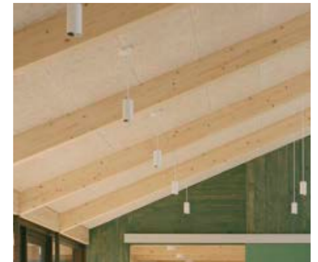
Interior - Simple plywood finishes with exposed beams
